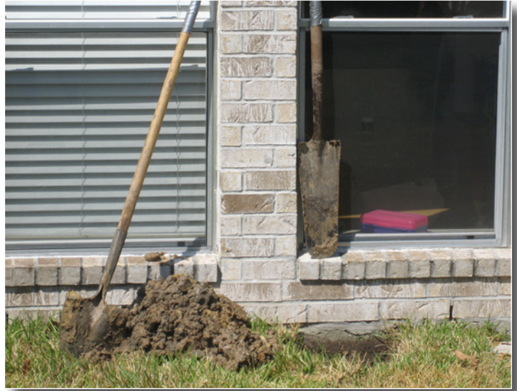
Figure 8. Picture showing the EX-3 excavation in the south wall of the foundation.
